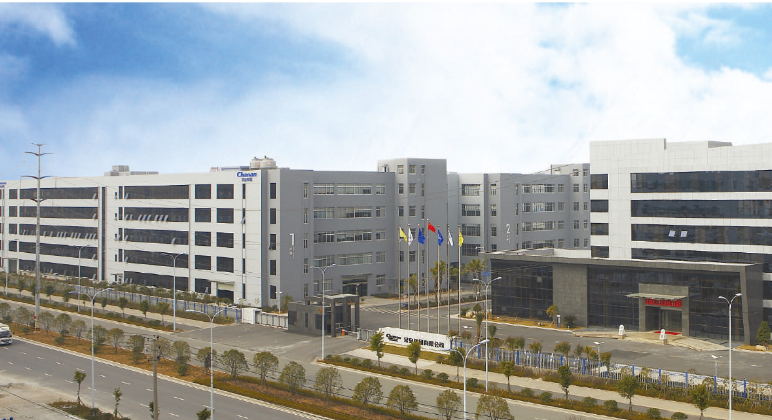
Changan Group Yueqing Economic Development Zone Industrial Park
